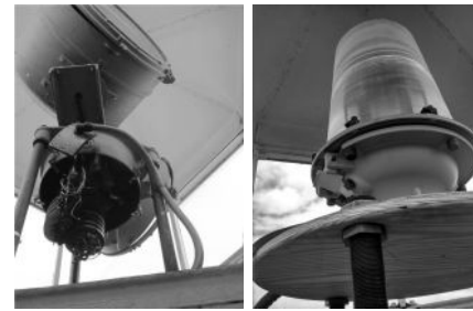
Image of old DCB 224 Aerobeacon (left) as compared to the Maxiluna 300 beacon.
