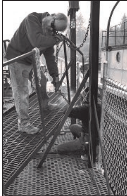
Tom Koehler and Bob Meier salvage the old gangplank and convert it into a safer walk way.
