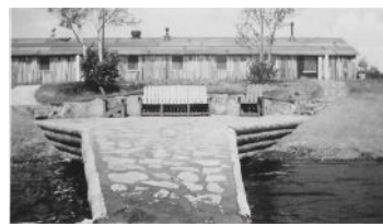
From Top: 00.2000.07 Construction of dock 00.2000.06 canoe dock completed, near Ely. Halfway Camp F-1, Company 704. c. 1935
